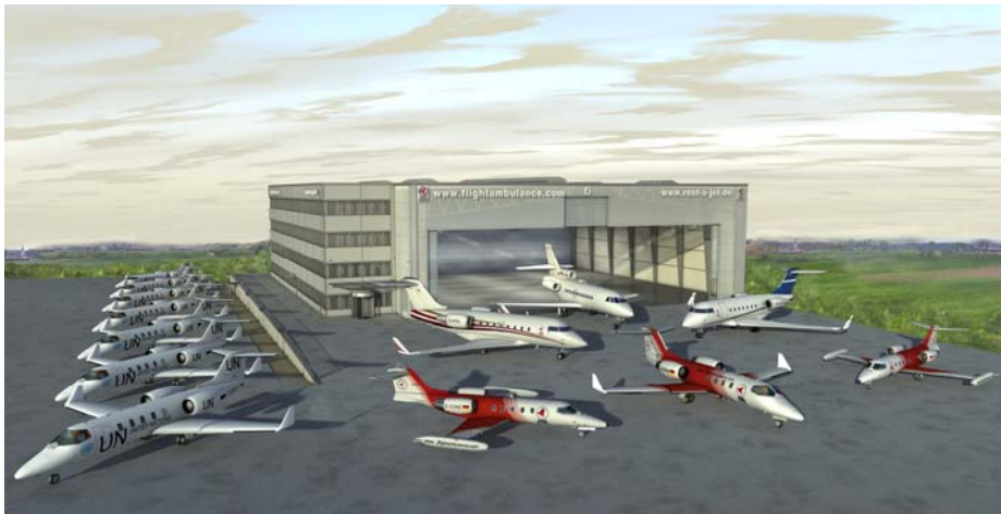
North View to FAI's Hangar
